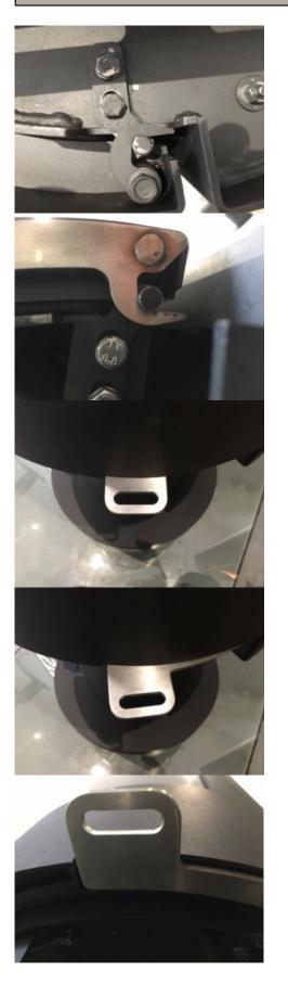
Top latch correctly fitted in closed position.
