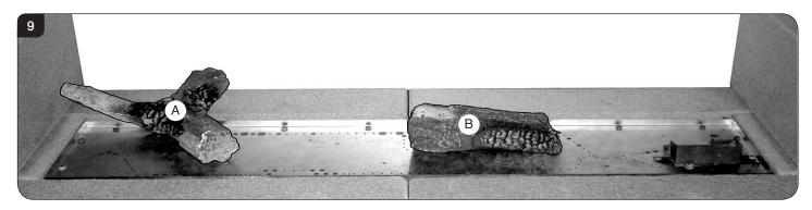
6.3 Use all the vermiculite to fill the burner tray between Logs A and B. Spread evenly across between the logs, so the whole burner is covered, see Diagram 10.
