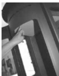
Place Top baffle in position against L shaped lugs leaving 5 cm gap at rear of stove.
